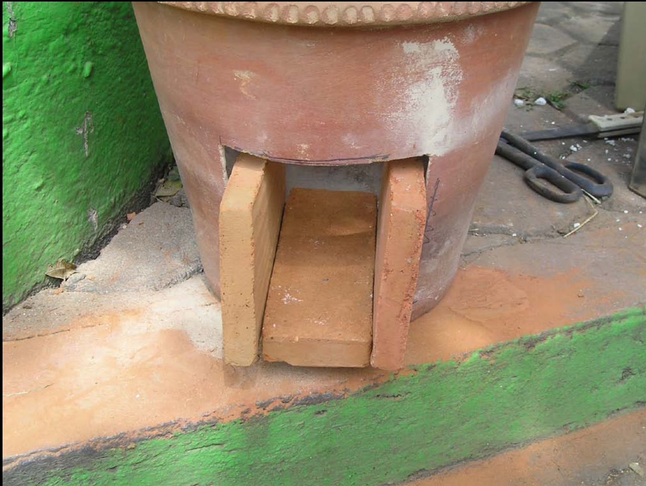
Flower pot rocket stove under construction
